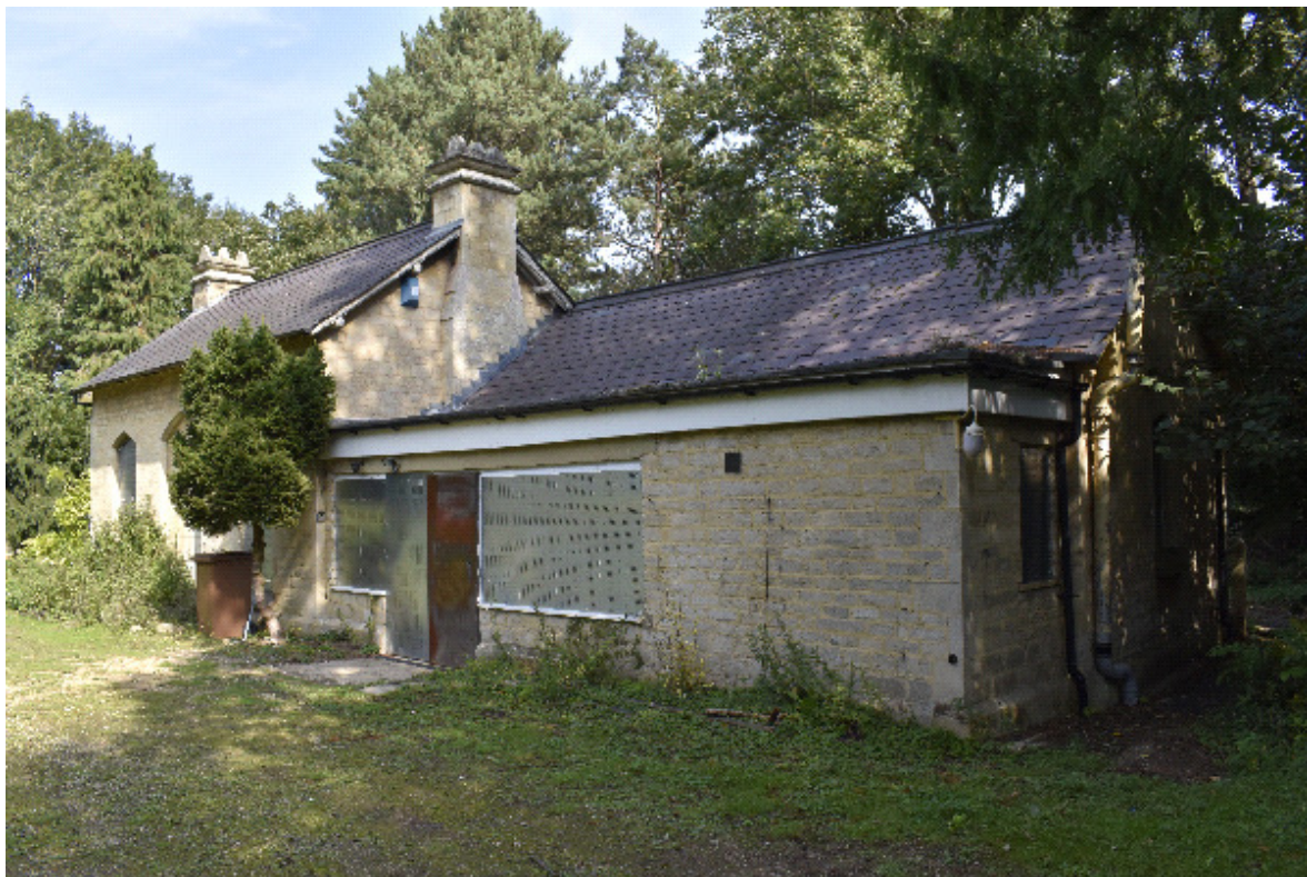
Photo 8 Former station, looking north-east
