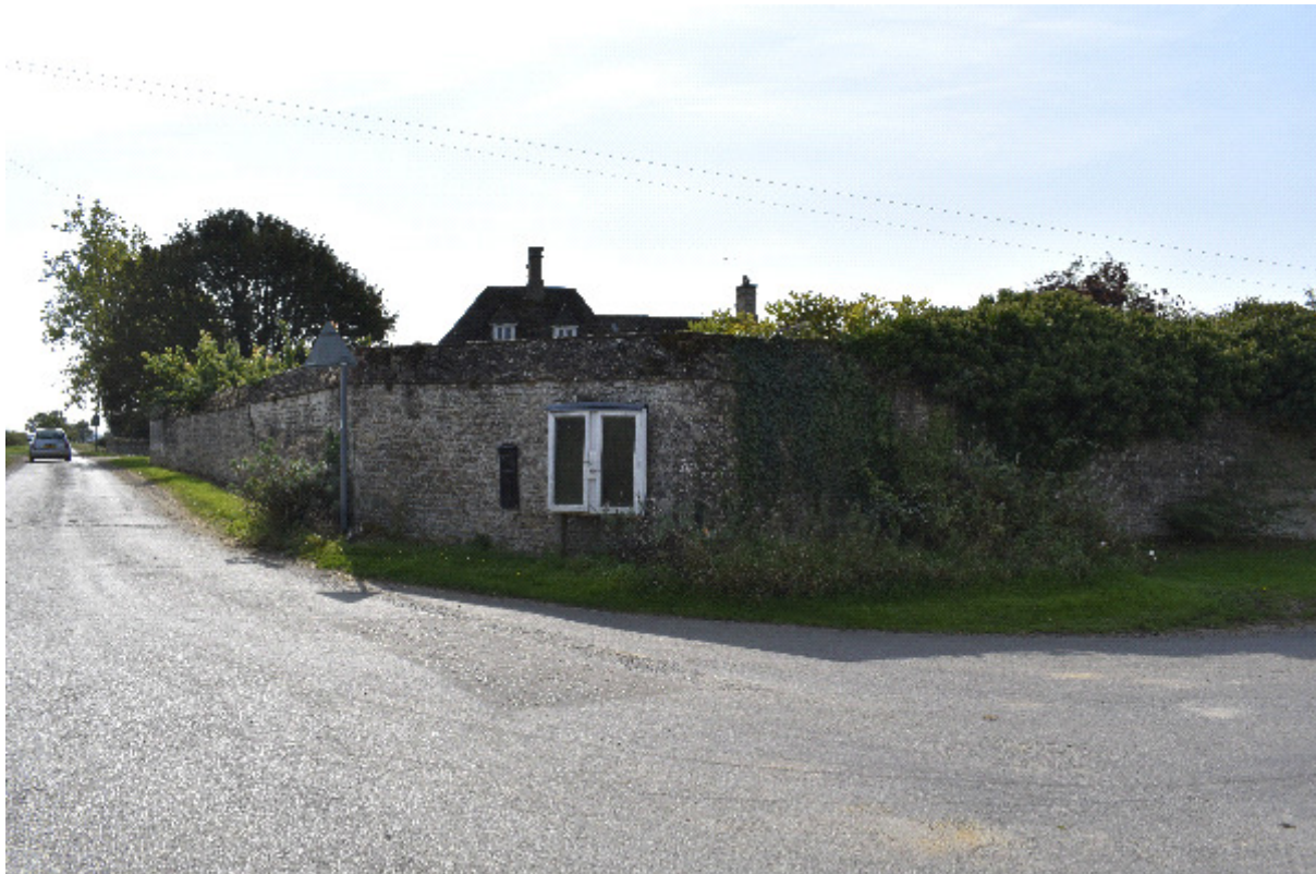
Photo 7 Model Farmhouse and wall, looking south-west
